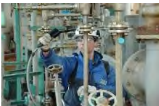
Figure 3.37: Leak concentration measurement
